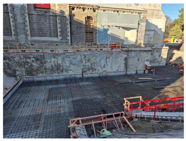
Construction workers have completed excavation for part of the 6-metre deep basement for the redeveloped Museum.
