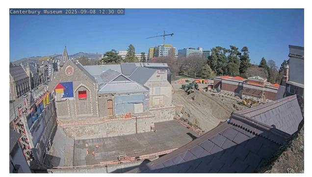
Part of the basement for the redeveloped Museum has already been excavated and is being prepared for the first big concrete pour.
