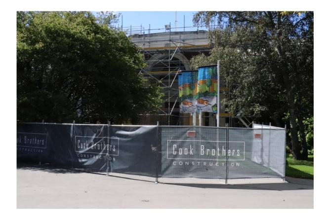
Scaffolding has been erected around the building (above) and in the near future, workers from Cook Brothers Construction will begin drilling vertical holes in the walls to house steel rods. This strengthening won't be visible, keeping the McDougall's heritage look intact.
