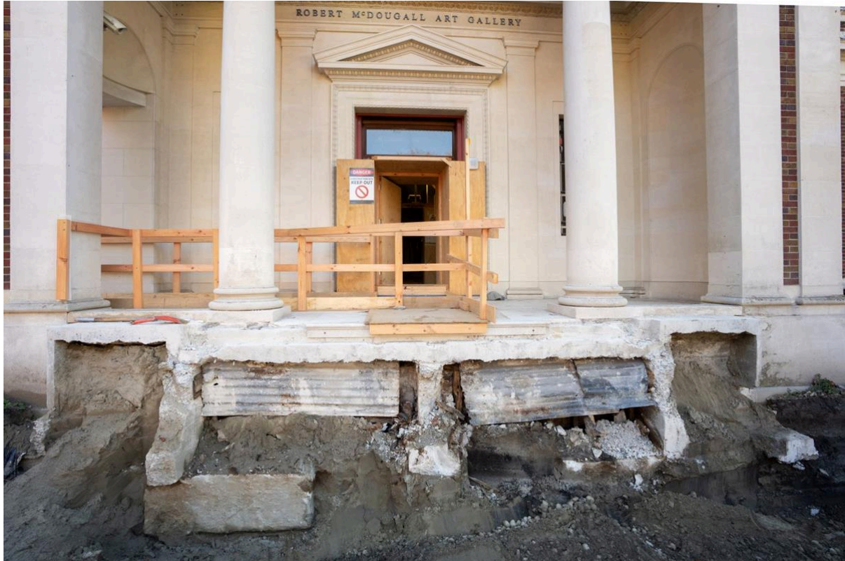
Contractors are preparing to demolish and excavate out the old Robert McDougall Gallery basement.
