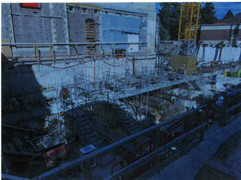
Zone 1 and 2 Base Isolators, Precast and Institu Grillage
