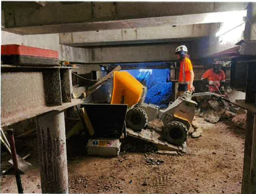
Basement demolition under the Robert McDougall Gallery
