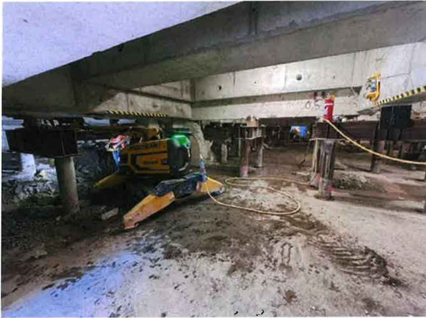
Basement demolition under the Robert McDougall Gallery
