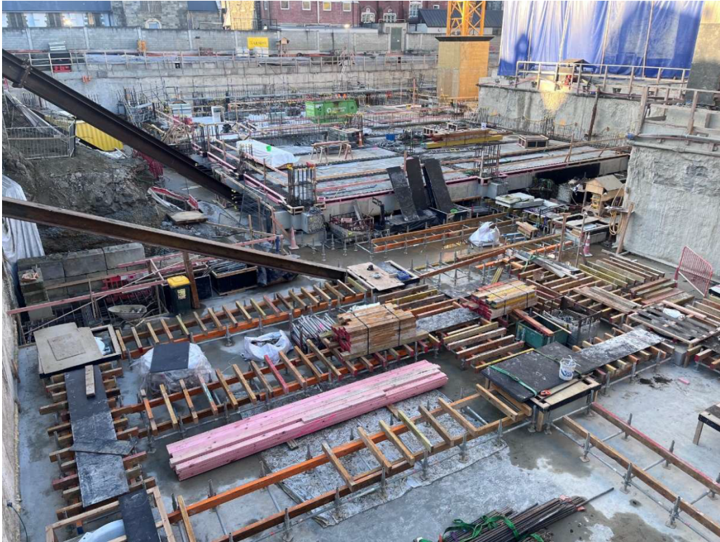
Zone 3 Base Isolators, Precast and Insitu Grillage
