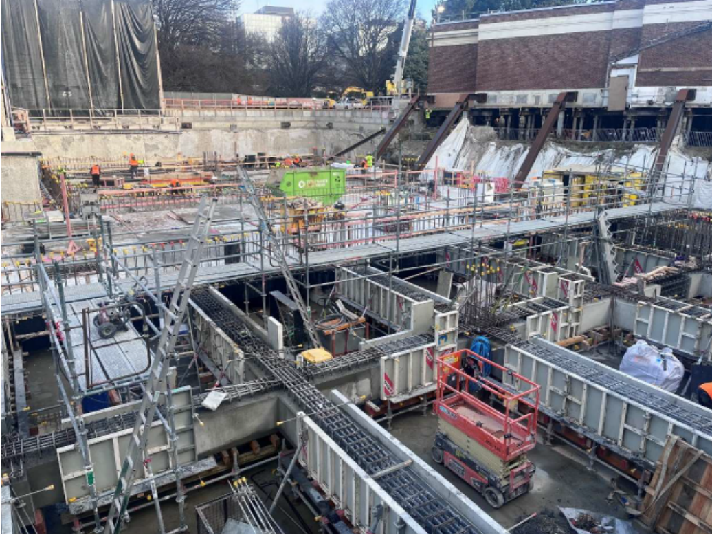
Zone 3-4 Flat Slab, Base Isolators, Precast and Insitu Grillage
