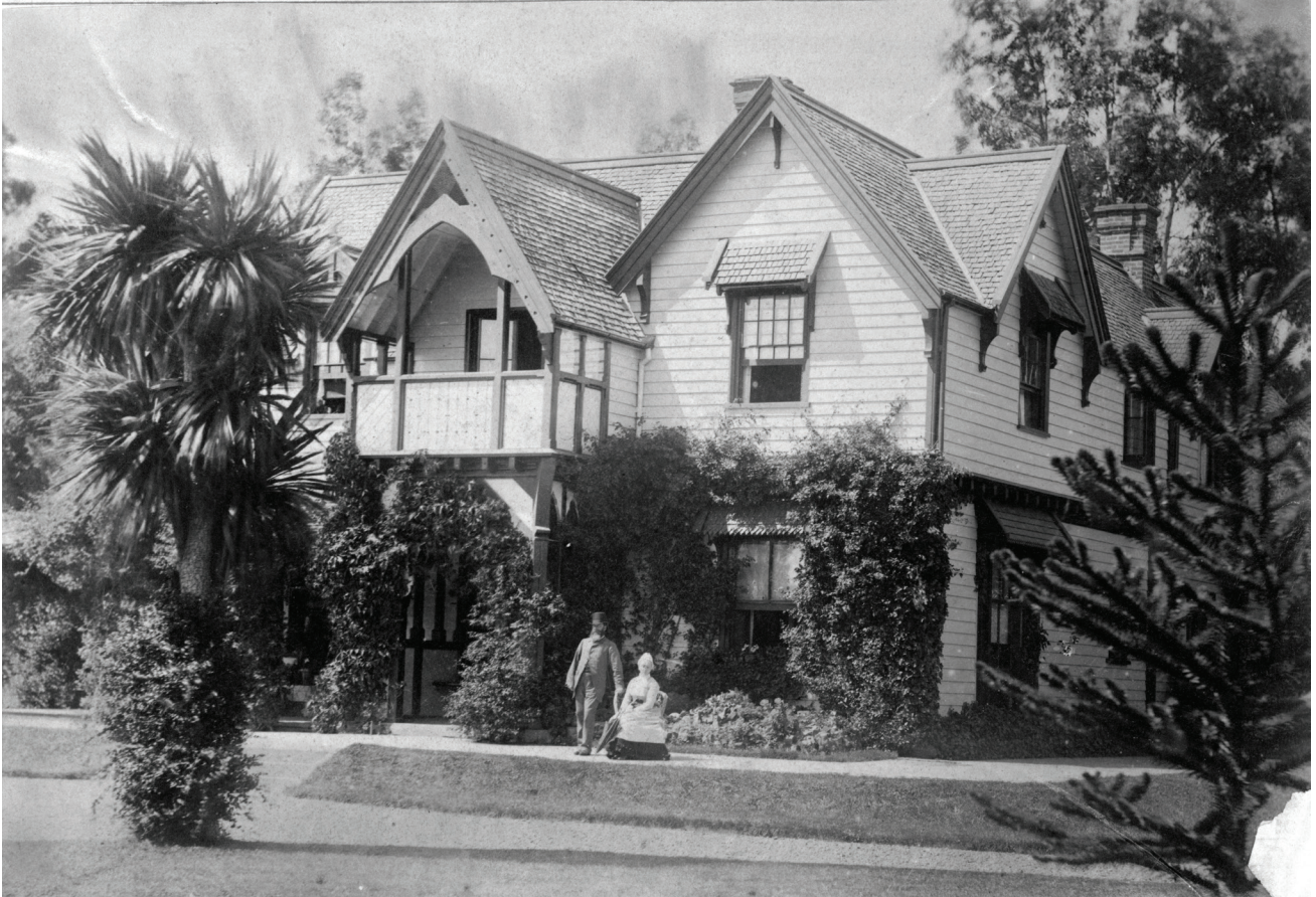
Figure 48. Ellen and William Reeves in front of their residence, Risingholme, c.1880. Canterbury Museum 19xx.2.2078
