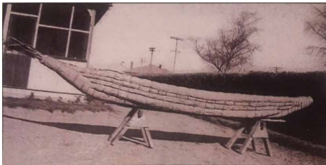
Figure 6. The almost completed mōkihi in Hugh McCully's backyard. McEvedy collection
