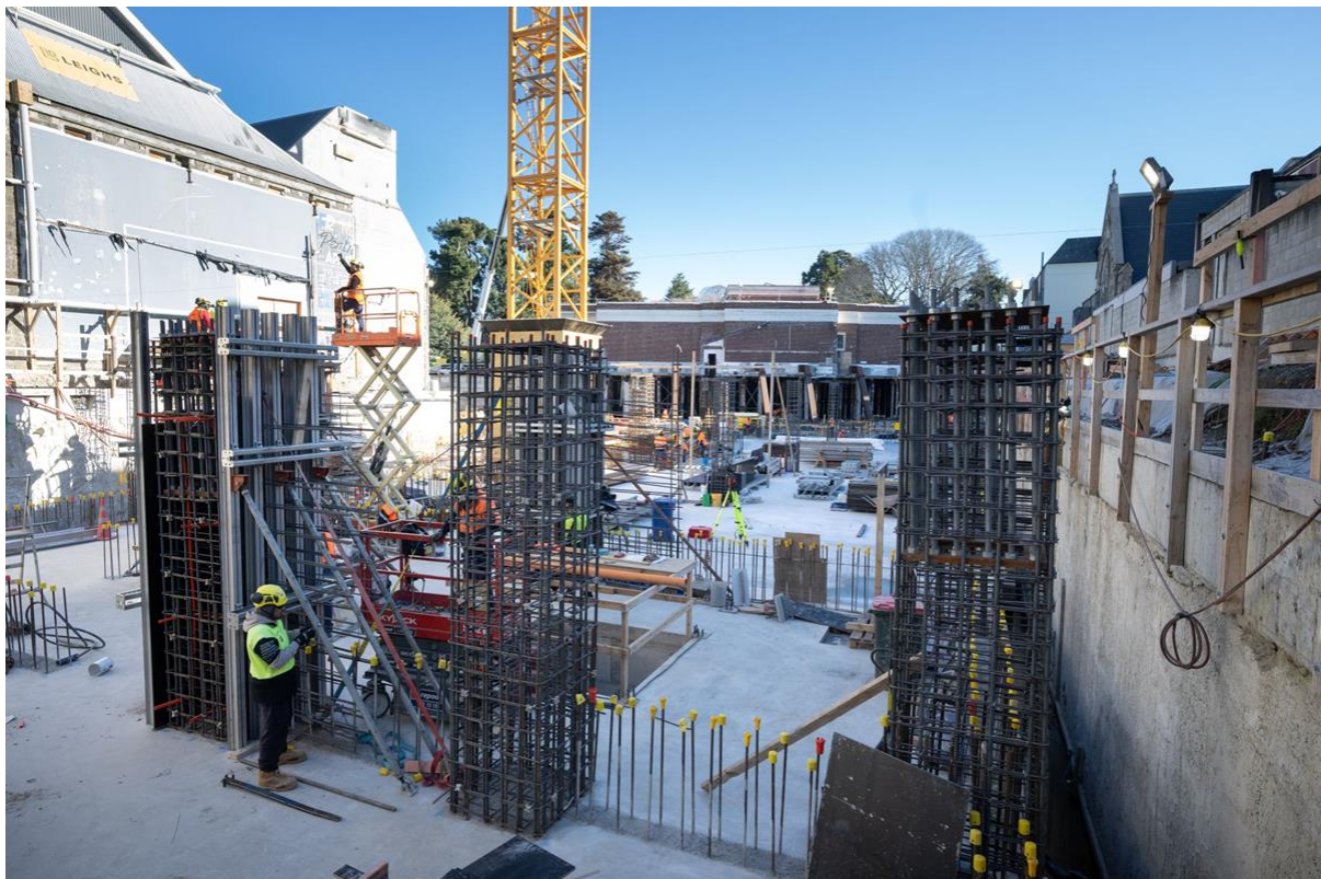
The columns in the new basement are starting to take shape.
