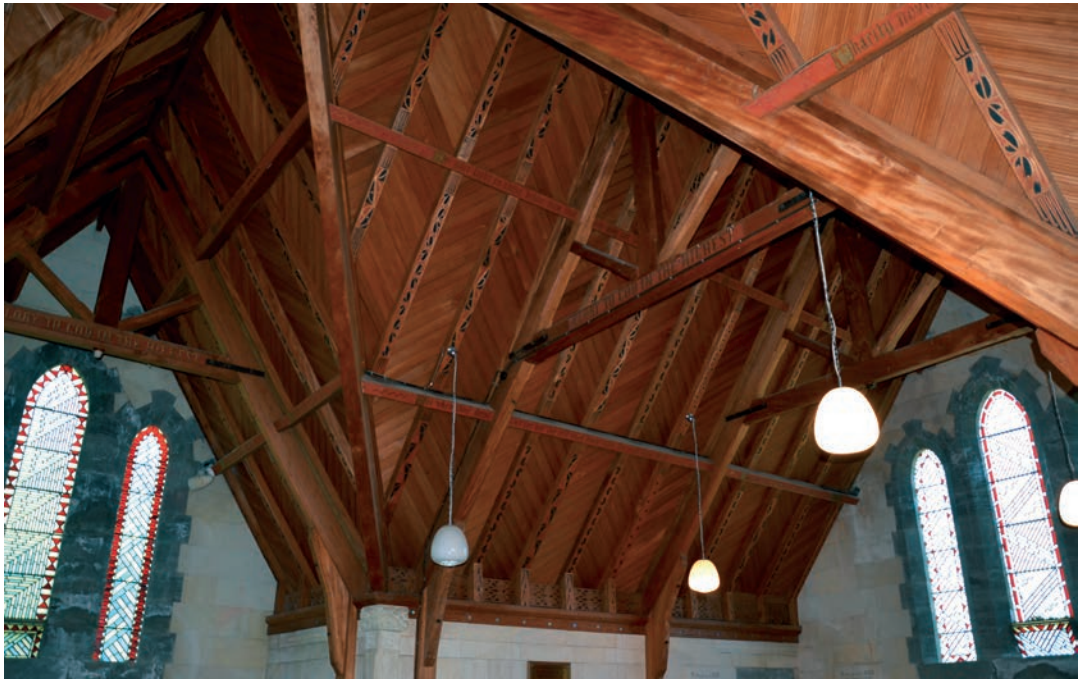
Figure 13. Roof space, St Luke's Church, showing rafters painted with kōwhaiwhai designs in red and black. Other timbers are painted with quotations from the Bible in gold lettering. Reeded panelling is fitted between the rafters. Photograph: D Smith, 2016
