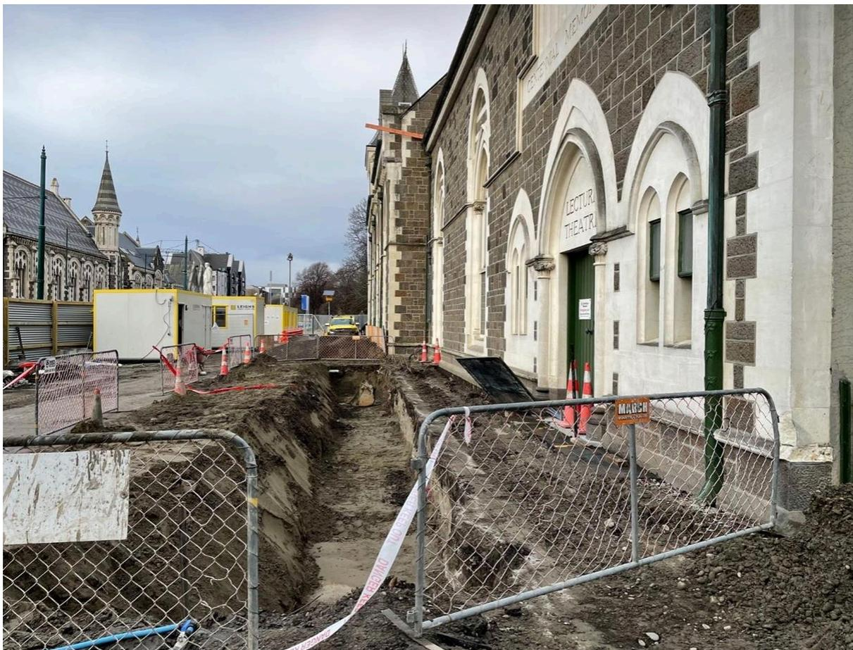
*The underground diaphragm wall that will enclose the new base-isolated basement has been installed in front of the Centennial Wing facade.*
