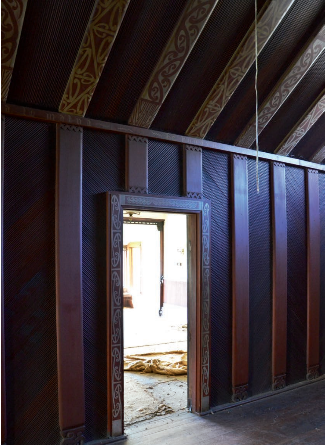
Figure 7. Hallway, Rehutai, showing kōwhaiwhai painting on heke (rafters) and around doorway. Note text in te reo Māori on cornice and the treatment of the poupou (pilasters). Photograph: D Smith, 2012
