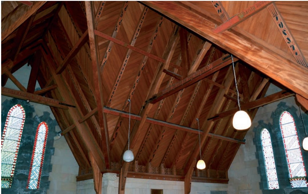
Figure 13. Roof space, St Luke's Church, showing rafters painted with kōwhaiwhai designs in red and black. Other timbers are painted with quotations from the Bible in gold lettering. Reeded panelling is fitted between the rafters. Photograph: D Smith, 2016
