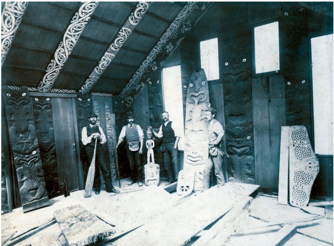
Figure 2. “Nearing completion”, a photograph of the decorated interior of the whare whakairo (carved house) Hau te Ana Nui o Tangaroa showing Pākehā carpenters posing with carvings from the frontage. Among the carved pieces yet to be attached are the koruru (carved face from apex of the maihi or bargeboards) surmounted by a tekoteko (carved figure) at the centre of the group of men. To the extreme right is a pare (carved lintel panel over a door or window) on its side. Photograph by John Bradley & Co, c. 1897, CMA 19XX.2.4905.
