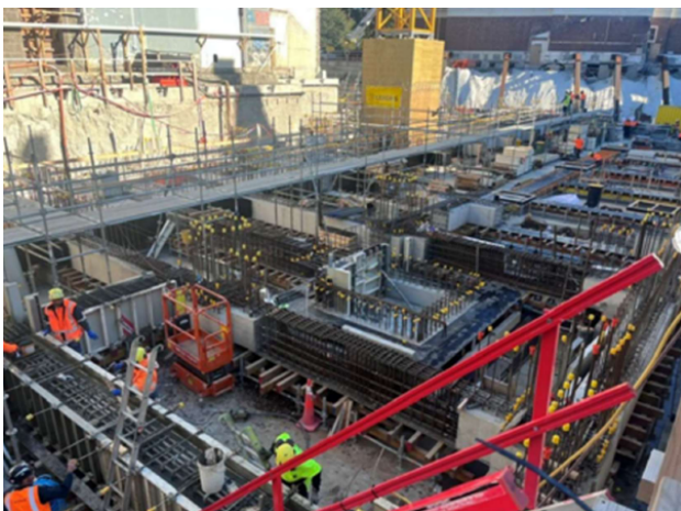
Zone 1-2 base isolators, precast and insitu grillage
