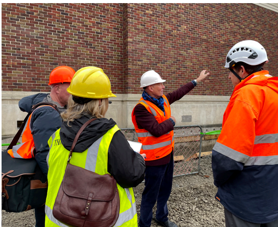
Museum Tūmuaki | Director Anthony Wright (middle) and Trevor Watt, Athfield Architects (right) talk to journalists at the Rolleston Avenue construction site.
