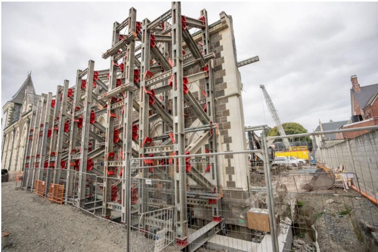
Top: Strengthening works on the Robert McDougall Gallery Above: Propping on the Rolleston Avenue grade 3 listed facade Front Cover: Exposed western end of 1882 building following demolition of the Roger Duff Wing Photographs taken February 2025.
