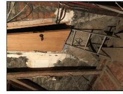
(5) View to the 1872 east wall with trachyte stone work, as seen from the 1877 building roof space.
