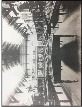
Historical photo showing the timber "double" trusses. (OHF)
