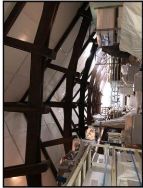
Original timber "double" trusses in space used for mammal storage. (OHF)
