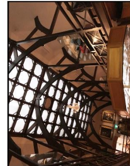
(4) Decorative arts area showing pointed arch trusses (OHF).
